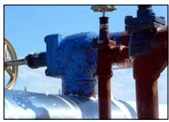
**RG-2400** LT is not "new" technology, it is new to the insulation industry and a breakthrough for corrosion control and prevention on piping systems, tanks and vessels under insulation. It is a non-drying compound easily brush/spray applied to pipes, fittings, valves, tanks and vessels. It's non-skinning and non-sag properties make it a permanent solution.
